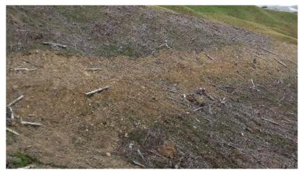
Figure 6: Example of a recontoured extraction track in a production forestry scenario. Note that full length trees were pulled along this track prior to recontouring.
